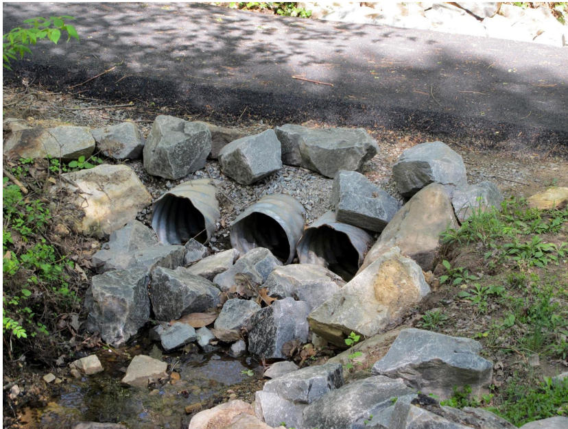
Culvert on Cuttermill Side
