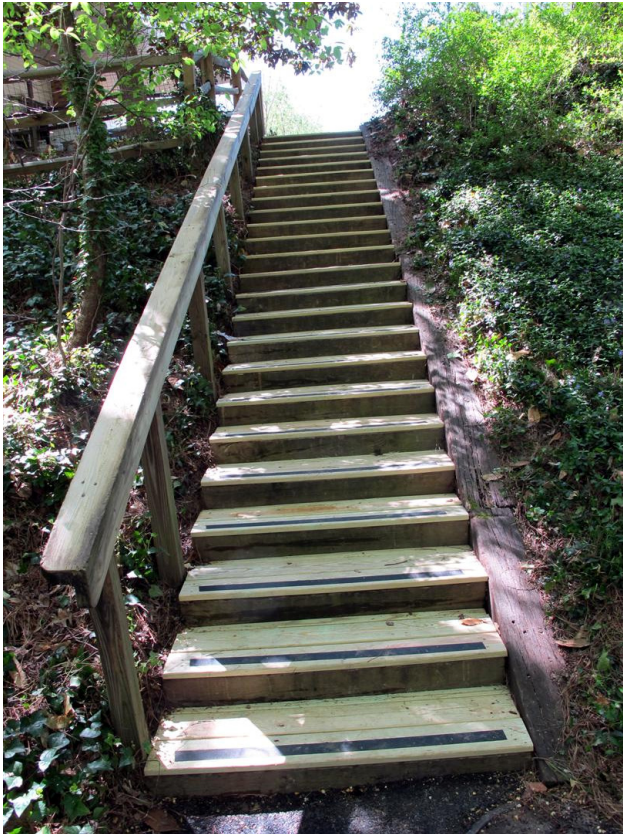
New Stair Treads
